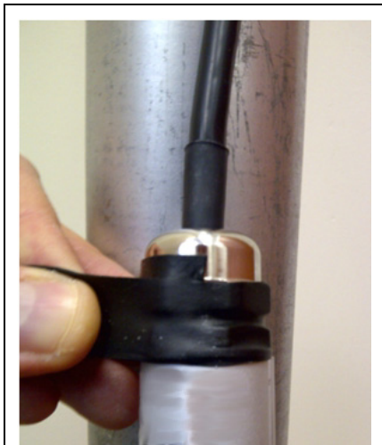
Figure 2-31: Applying sealant tape to an external connection
