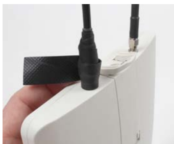
Apply sealing tape - 2
